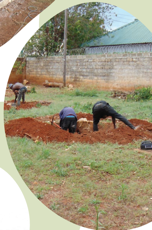
Solid level base being laid for the containers to be placed
