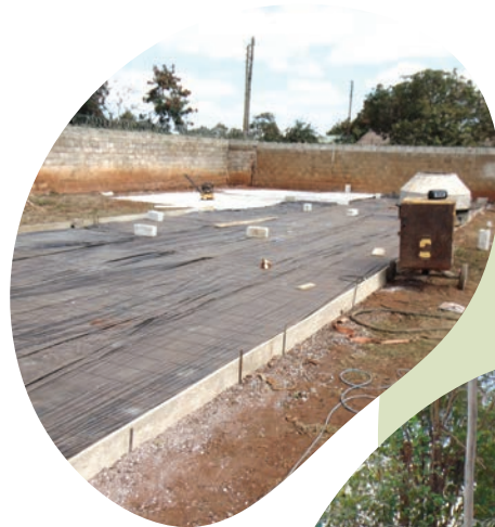
Solid level base being laid for the containers to be placed
